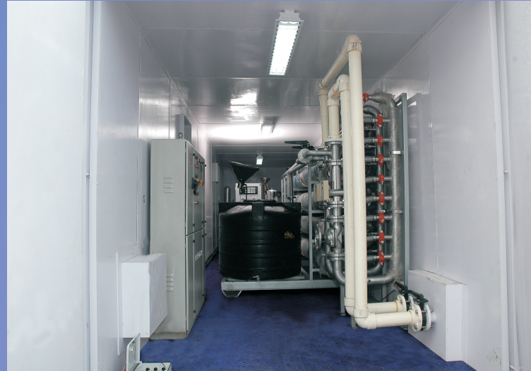
Internal view - Container
