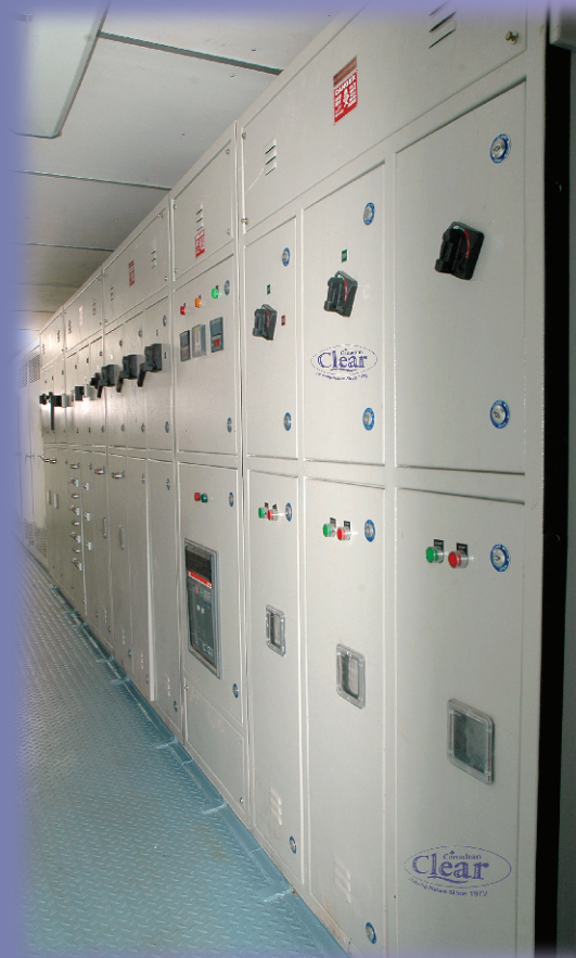
VFD & Electrical Panel - Containerized.
